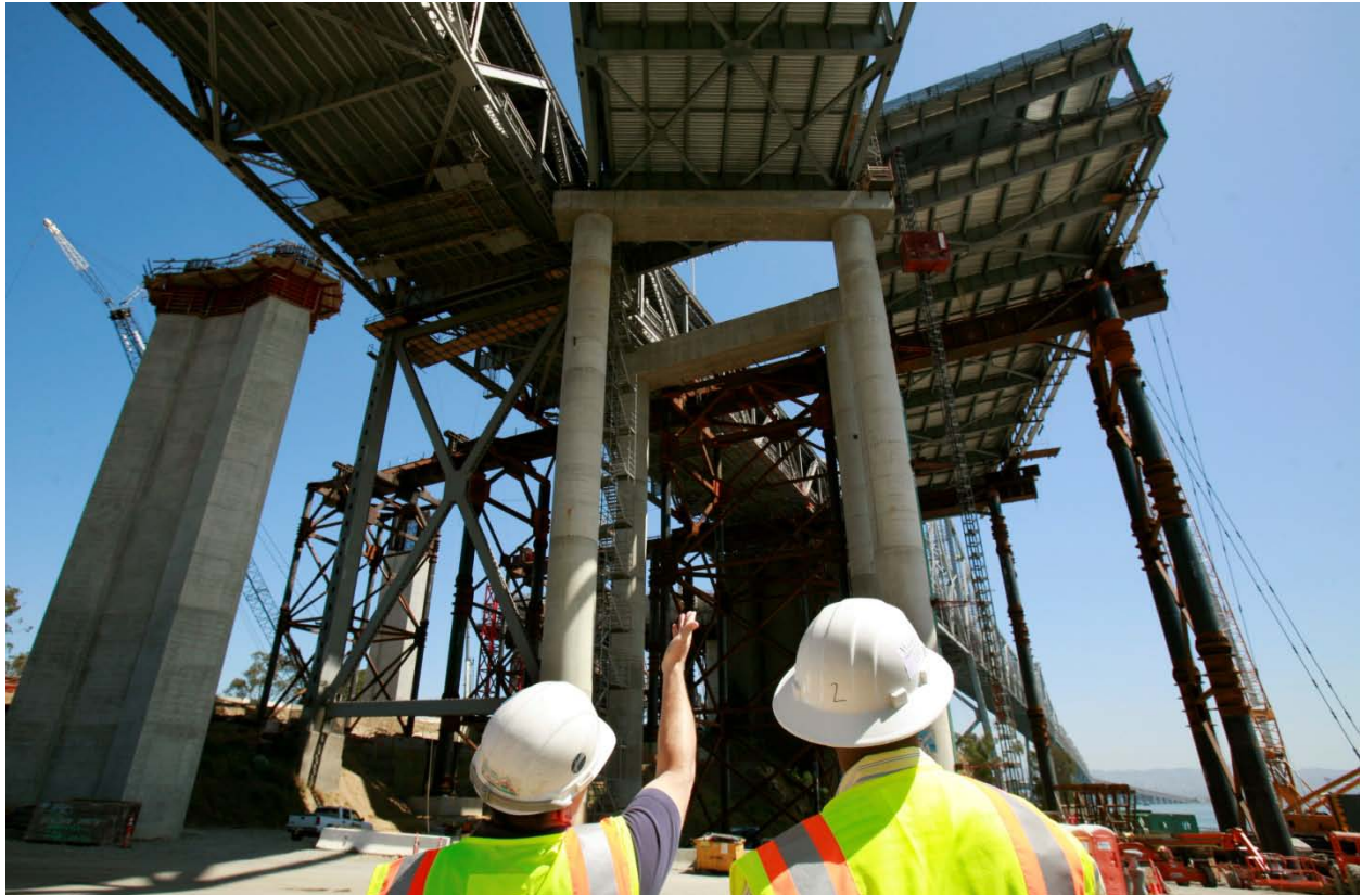
Reuters/ Robert Galbraith – A CalTrans worker displays a new section of roadway on the San Francisco Bay Bridge.
